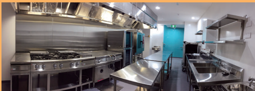
TIH's new kitchen facility
